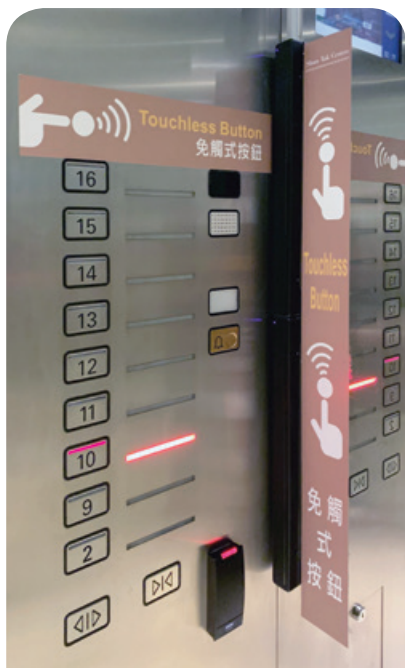
Installation of touchless lift control panels 安裝免觸式電梯控制面板
