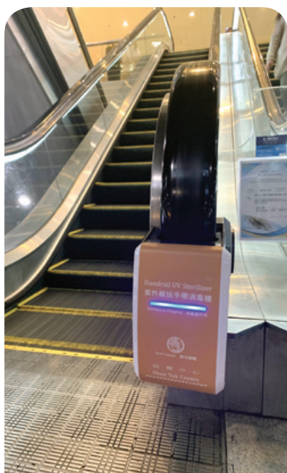
UV light escalator handrail cleaners installed to inhibit germs and viruses on escalator handrails 在扶手電梯安裝紫外線消毒殺菌器以抑制細菌和病毒滋生
